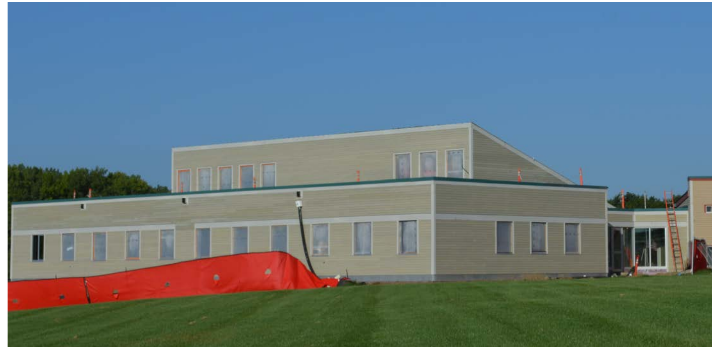
ENREC Christenson Building Addition construction underway.
