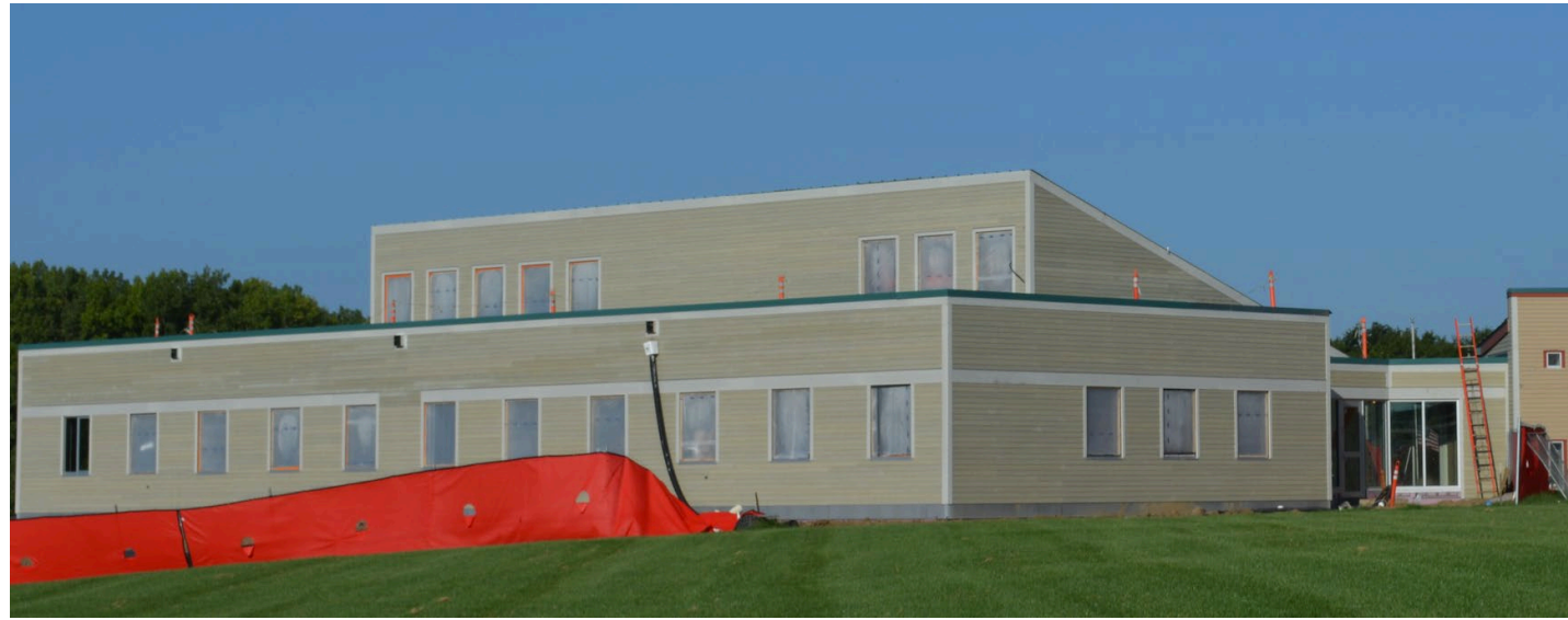
ENREC Christenson Building expansion
